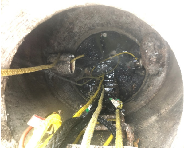
Collection manhole outside wetwell prior to coating.
