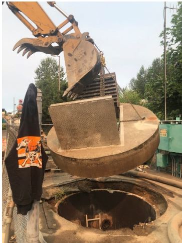
Removal of old wetwell hatch.
