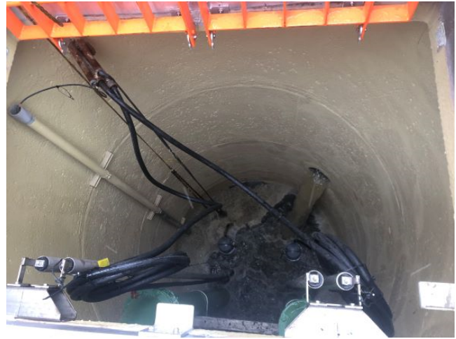
Finished wetwell upgrade.
