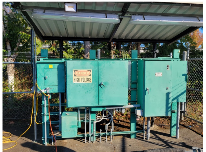
New roofing over controls area.
