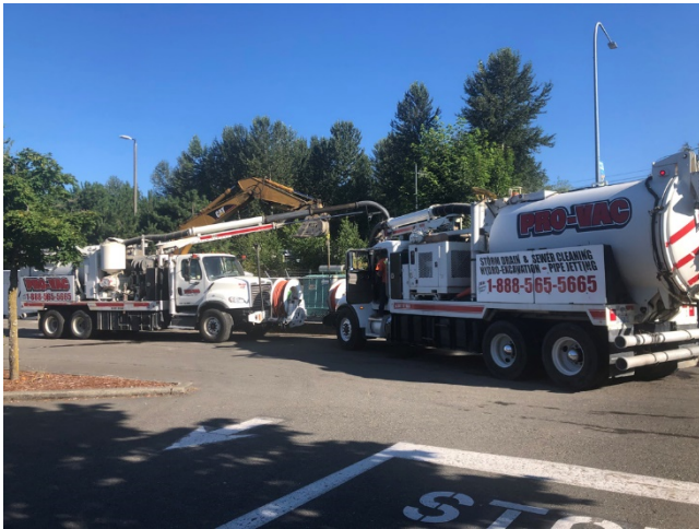
Vacuum trucks on site for valve vault upgrade.
