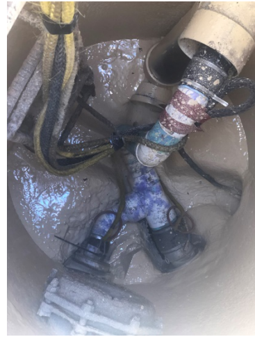
Collection manhole after new coating and prior to bypass piping removal.
