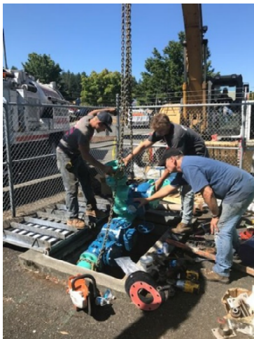
New piping installing in valve vault.
