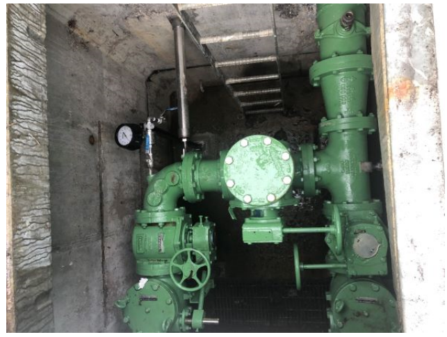
Finished valve vault upgrade.
