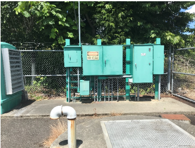
Controls area of site prior to construction.
