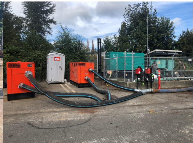
Bypass pumping during construction.
